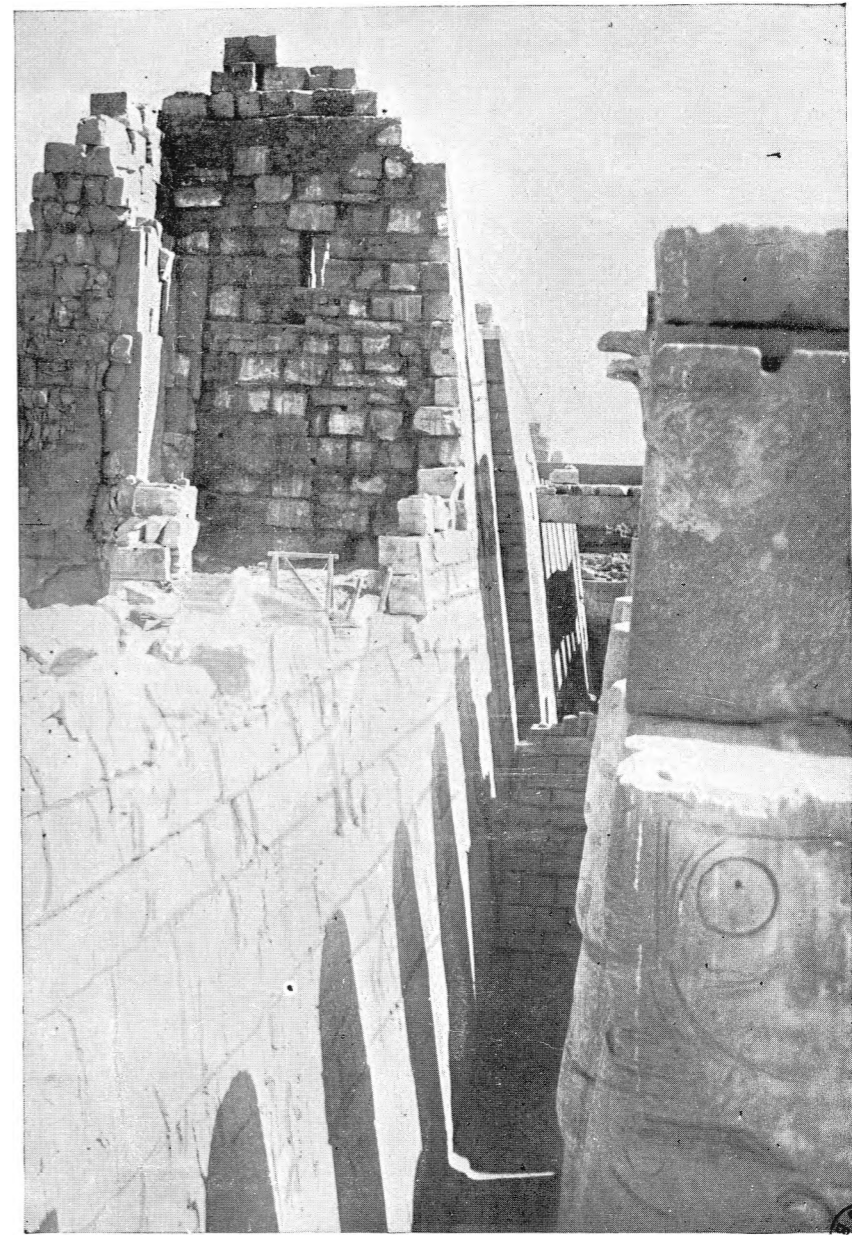
The Second Pylon after the restoration.
