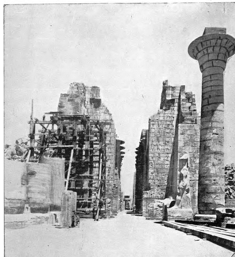
The Second Pylon after the restoration,
