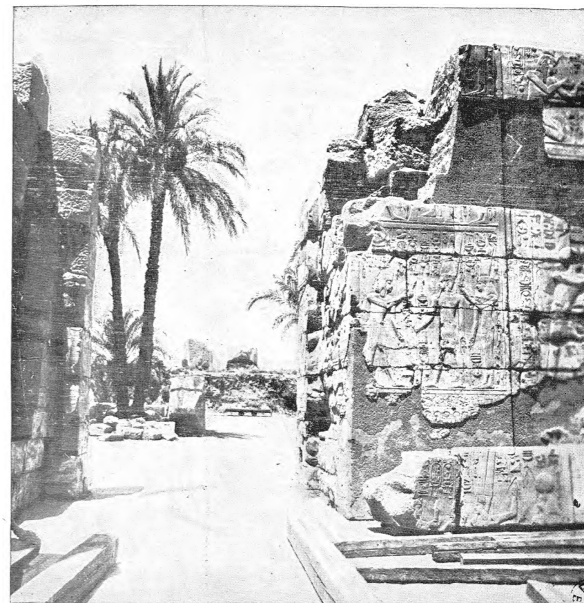
The wall of the Hypostyle Hall before the restoration.
